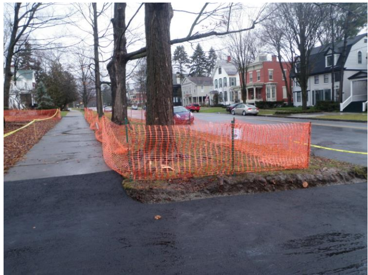
Image 5: This is an example of tree protection at a construction site. While the trees are protected and the disturbed roots were not torn, but cleanly cut; it could be argued that all disturbance to these trees could have been avoided if the site was accessed from the rear alley only.
