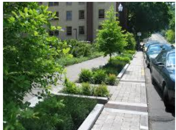
Image 10: NYC is giving trees a better growing environment by increasing rooting volume and integrating stormwater management systems with the planters.
