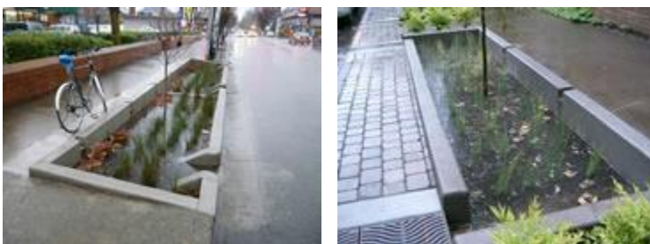
Image 11: In Portland Oregon, Stormwater infrastructure and street trees are integrated in large planters.
