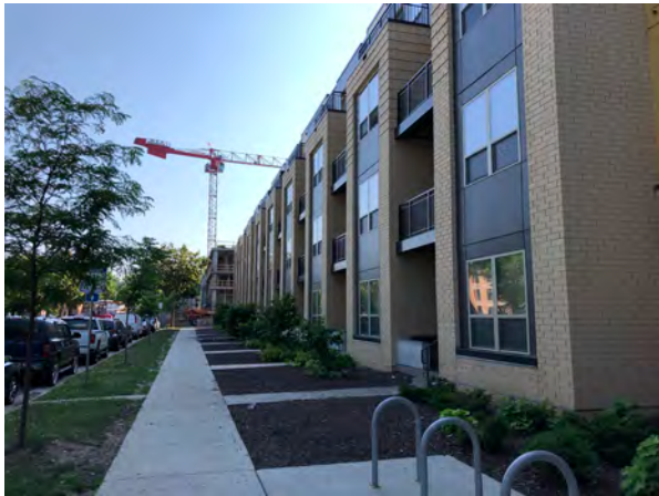
Ground floor residential units facing the street must have their own entrances from the sidewalk.
