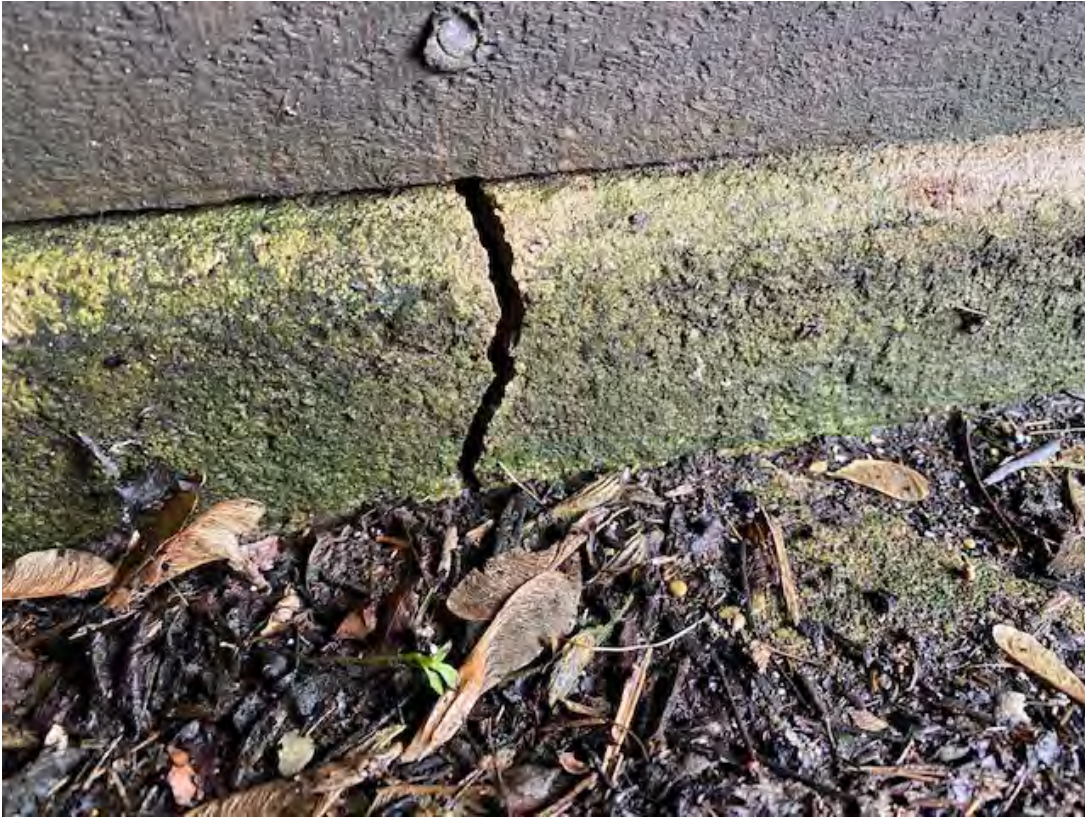
Foundation cracked
