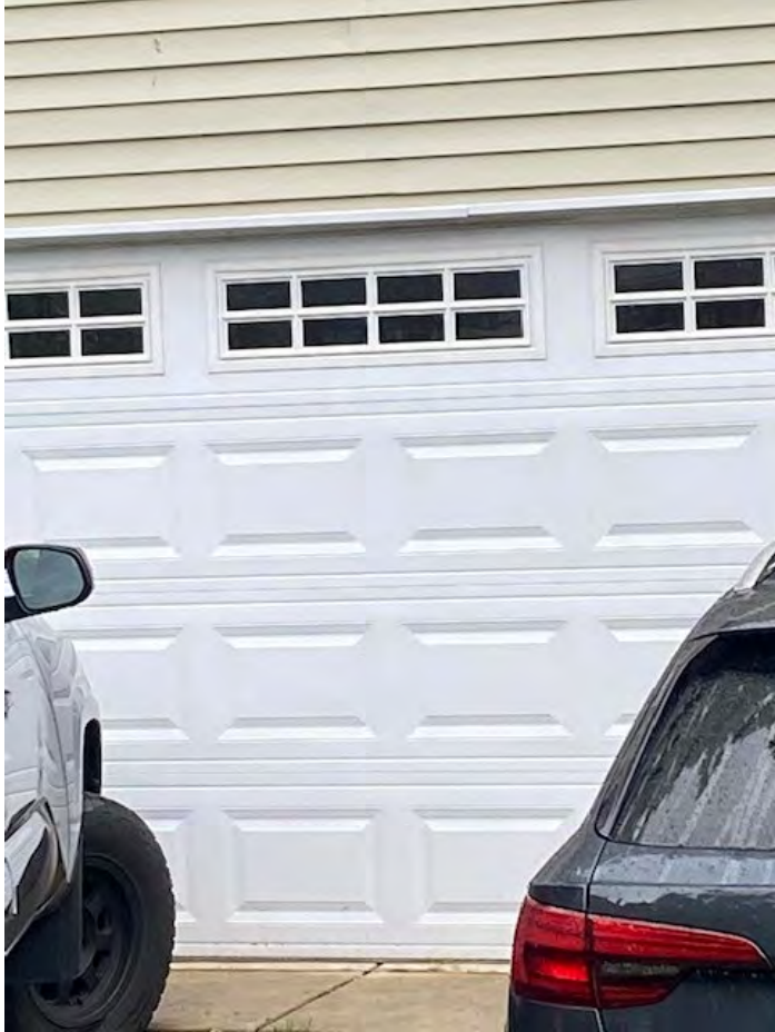
Existing garage door at 1323 Spaight St.
