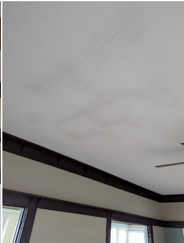
Images of first floor settling and cracking at original building living spaces.
