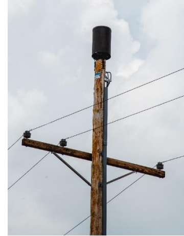
Small cell antenna
