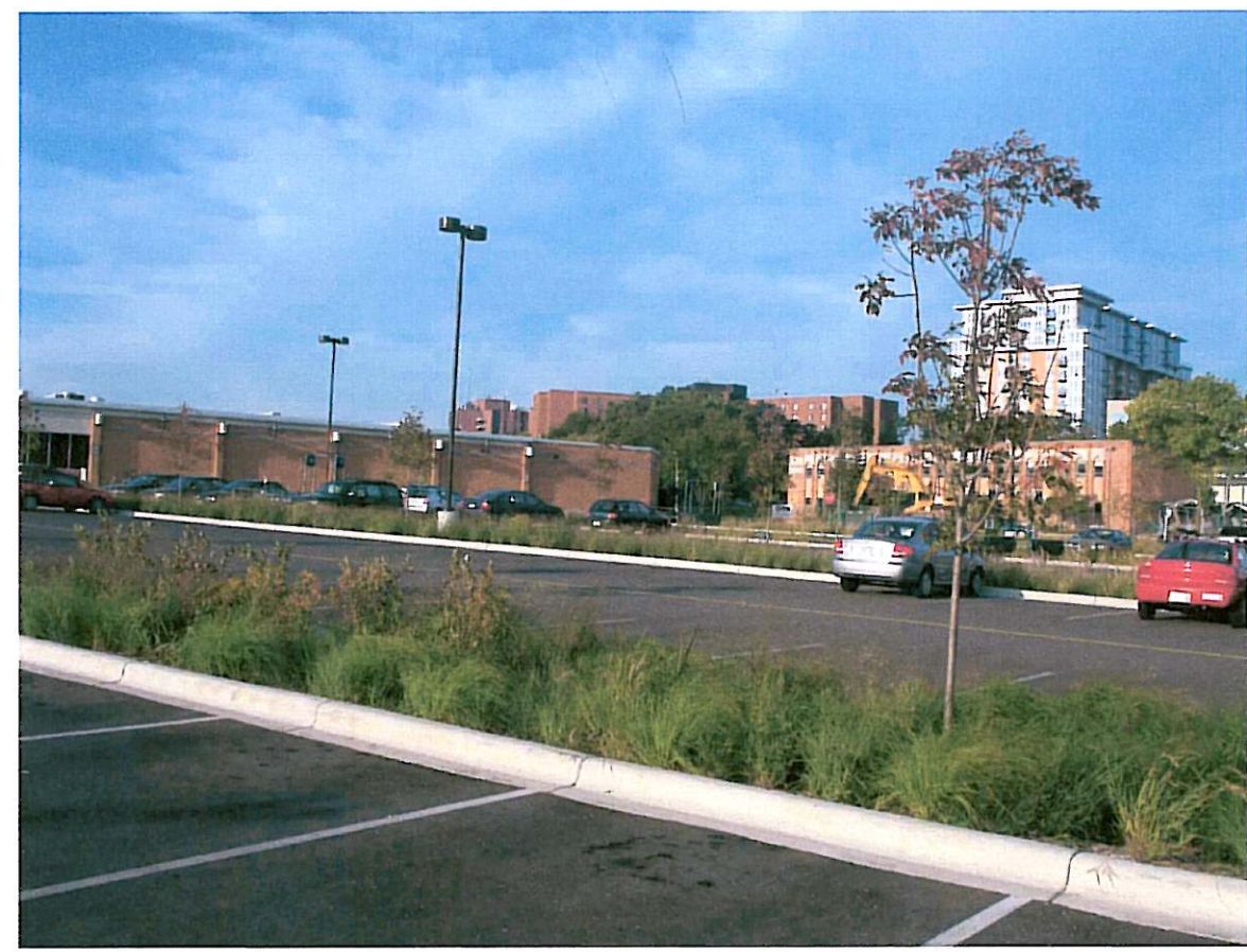
Installed Bioswale Planting
