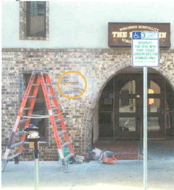
View of one probe location on the Carroll Street façade. October 1, 2015.
