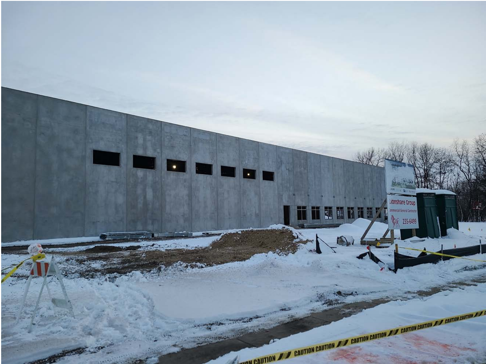
Illingworth-Kilgust Mechanical – 4701 Tradewinds Parkway (Currently under construction by MPI/Lionshare Group)
