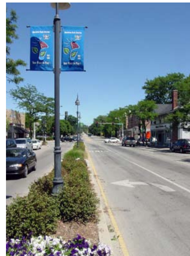
Figure I-3: Traffic Calming: Landscaped Portion of a Pedestrian Refuge Median in Downtown Glenview, Illinois
