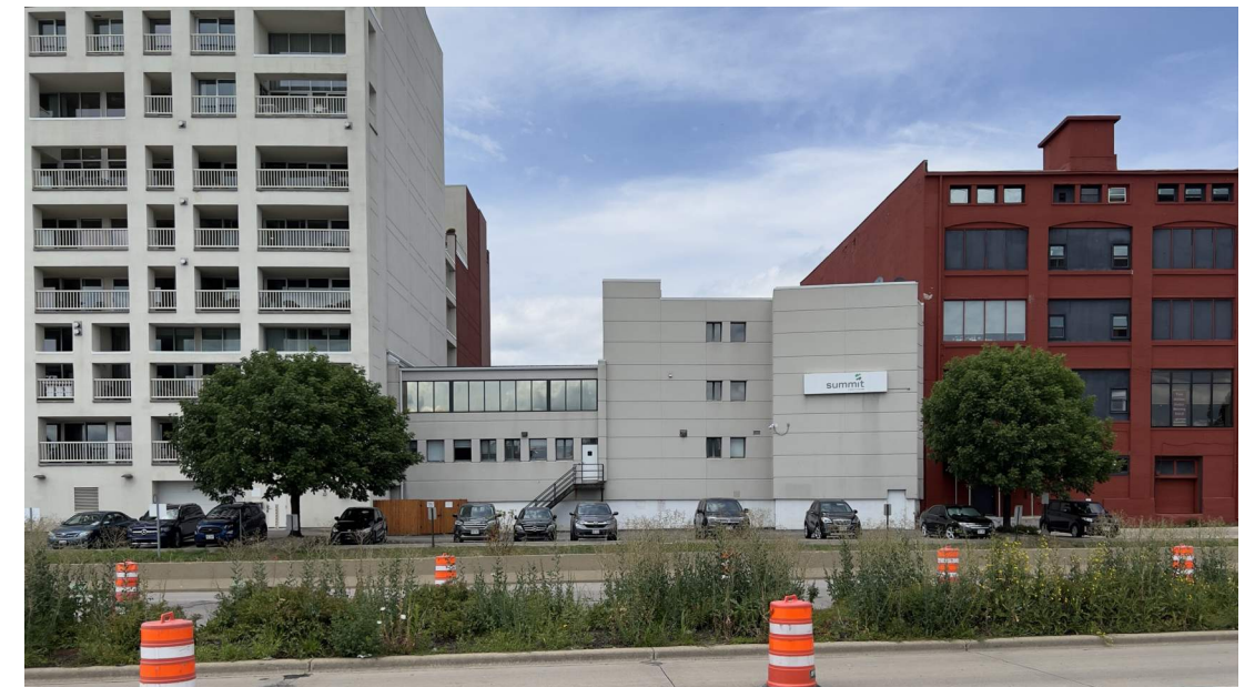
EXISTING JOHN NOLEN BLVD. FACADE
