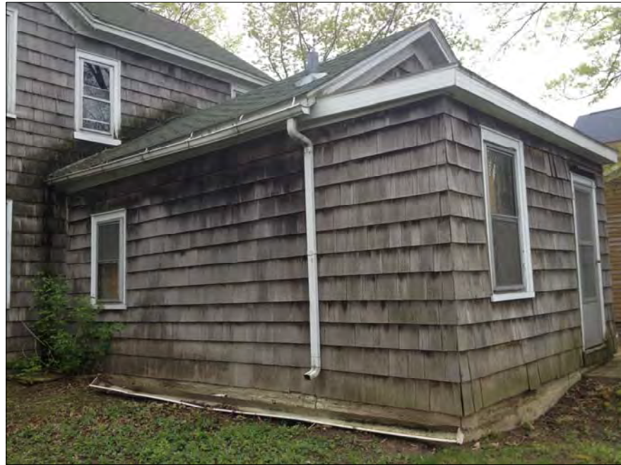
CLOSE-UP OF EXISTING ONE STORY ADDITION
