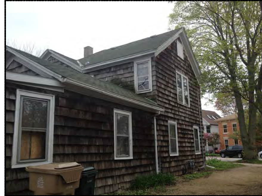
CLOSE-UP OF EXISTING ONE STORY ADDITION
