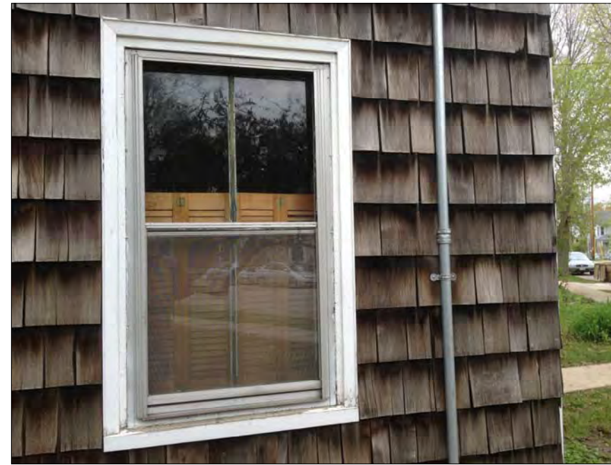
CLOSE-UP OF EXISTING WINDOW
