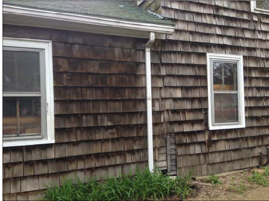
CLOSE-UP OF EXISTING ONE STORY ADDITION
