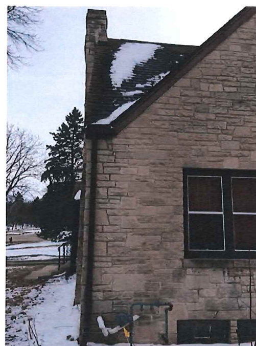
Northeast Corner & Chimney
