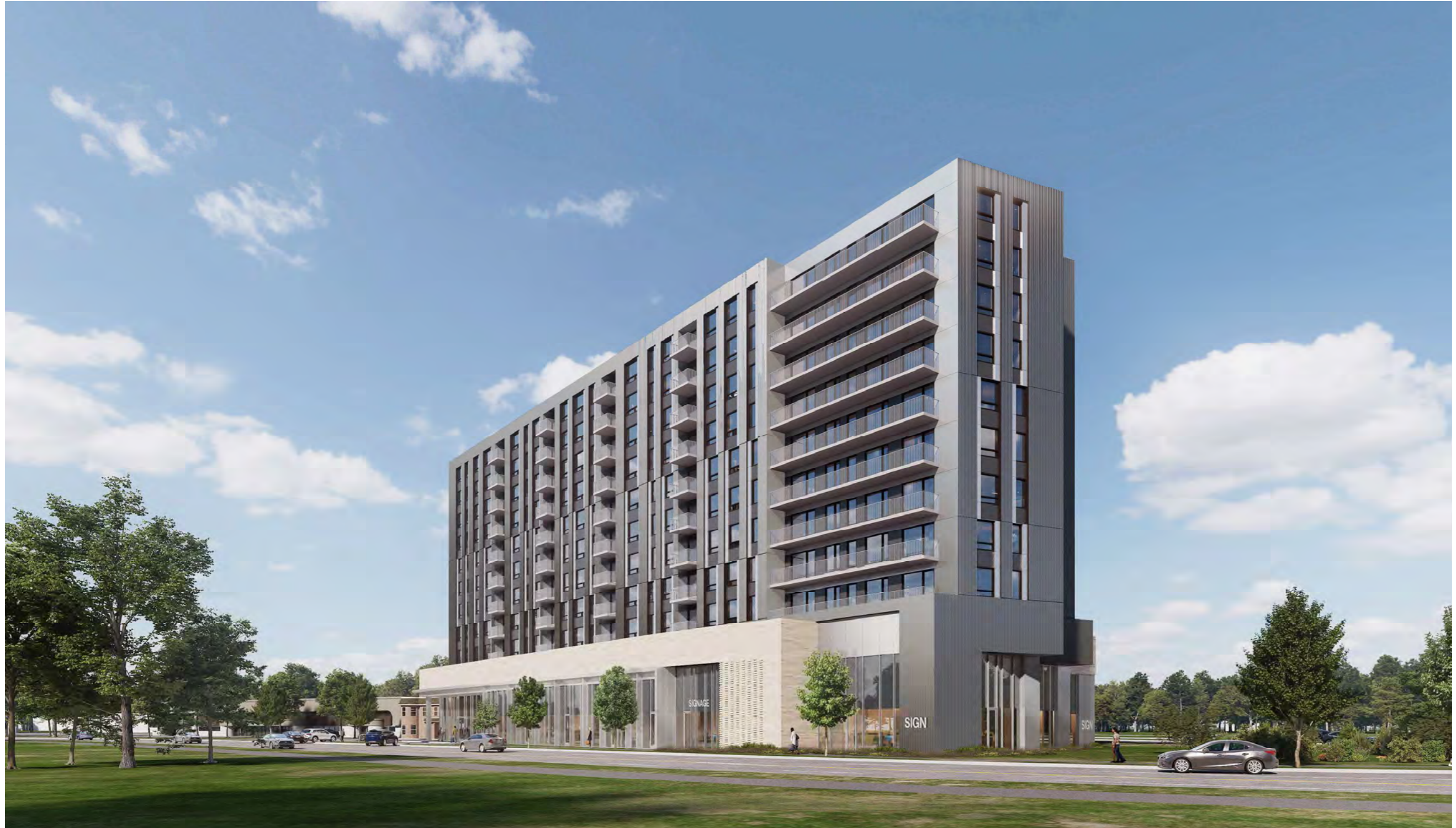
View from East Olin Avenue looking north
