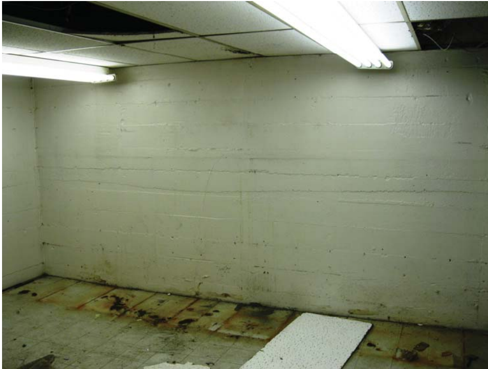
Photo 1 – Concrete basement wall at Mifflin / Fairchild corner
