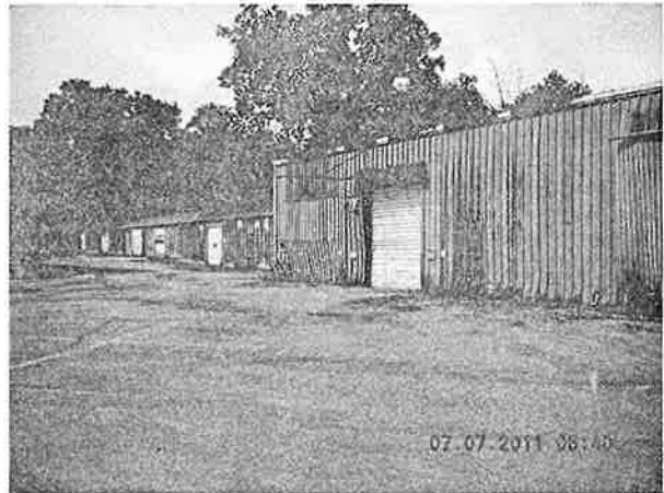
5119 UNIVERSITY AVENUE, FORMER "GREY SHED"
