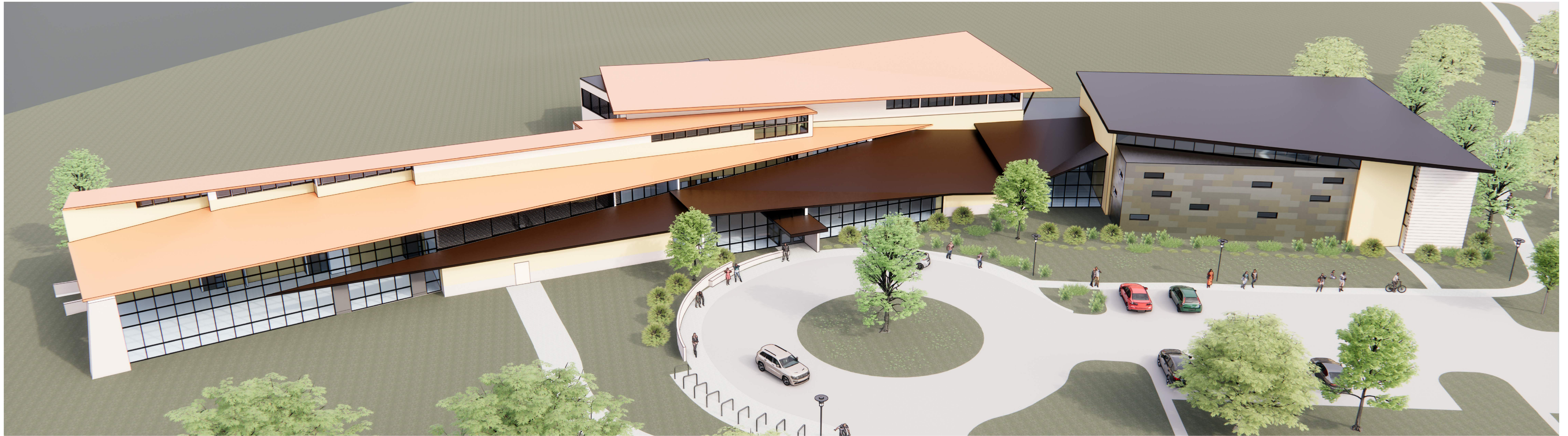
OVERHEAD VIEW FROM SOUTH
