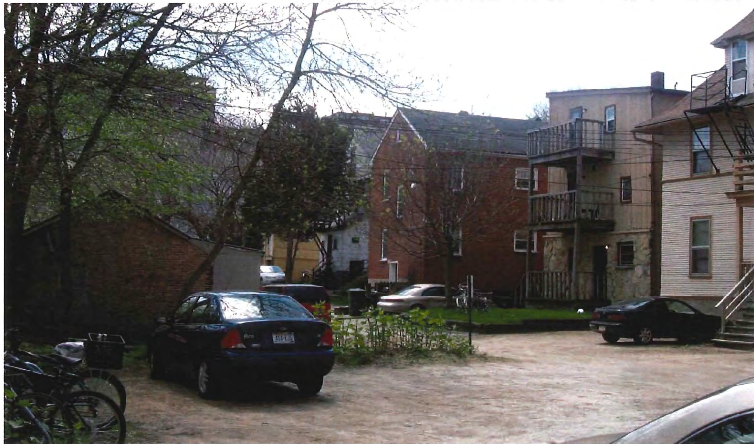
View from the North East (Rear) of 119, 123 & 125 North Butler
