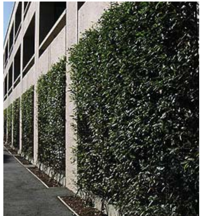
vegetative screening/green wall - screening parking structure
