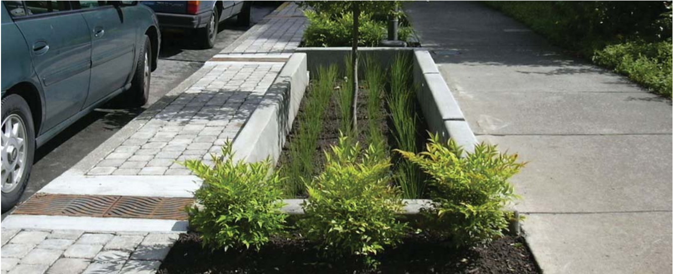
stormwater management - flow through planter curb
