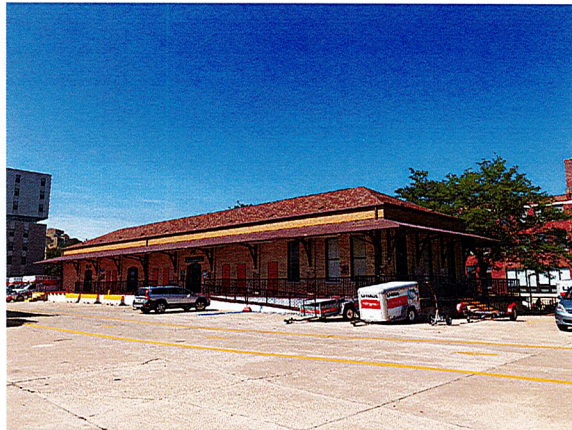
View of building at Corner of Washington and Bedford.
