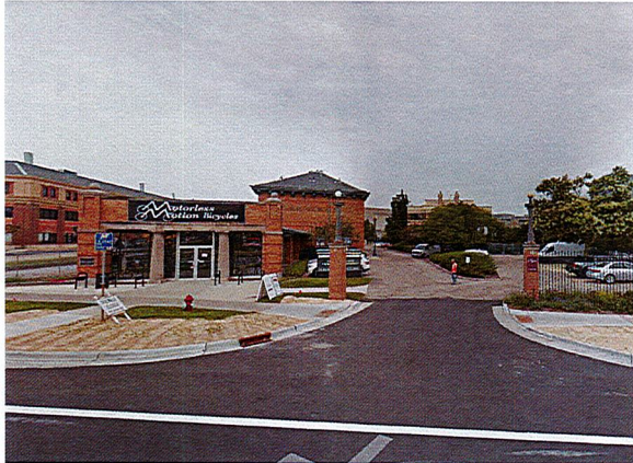
View of building directly adjacent and Southwest of Site.
