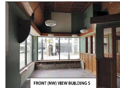
FRONT (NW) VIEW BUILDING 5
