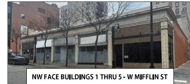
NW FACE BUILDINGS 1 THRU 5 - W MIFFLIN ST
