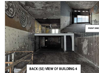
BACK (SE) VIEW OF BUILDING 4
