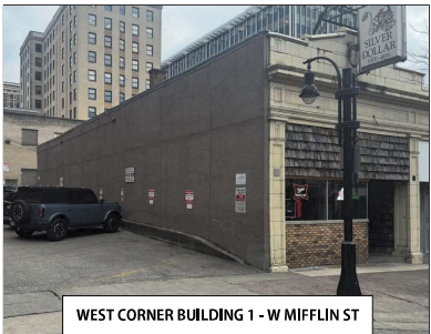
WEST CORNER BUILDING 1 - W MIFFLIN ST
