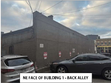
NE FACE OF BUILDING 1 - BACK ALLEY
