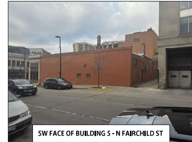
SW FACE OF BUILDING 5 - N FAIRCHILD ST
