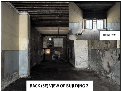
BACK (SE) VIEW OF BUILDING 2
