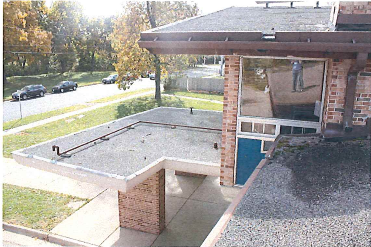
D1 A110 VIEW FROM ROOF TOWARDS LOCATION OF ADDITION
