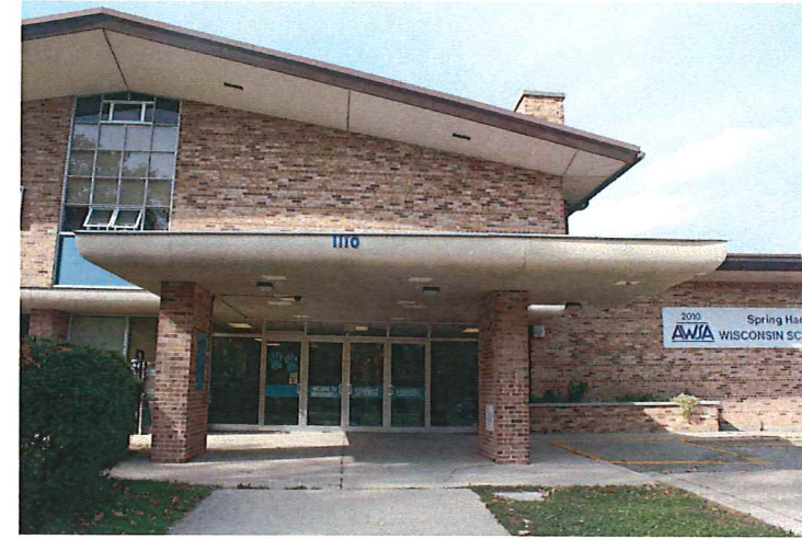
B5 A110 VIEW TOWARDS EXISTING MAIN ENTRY
