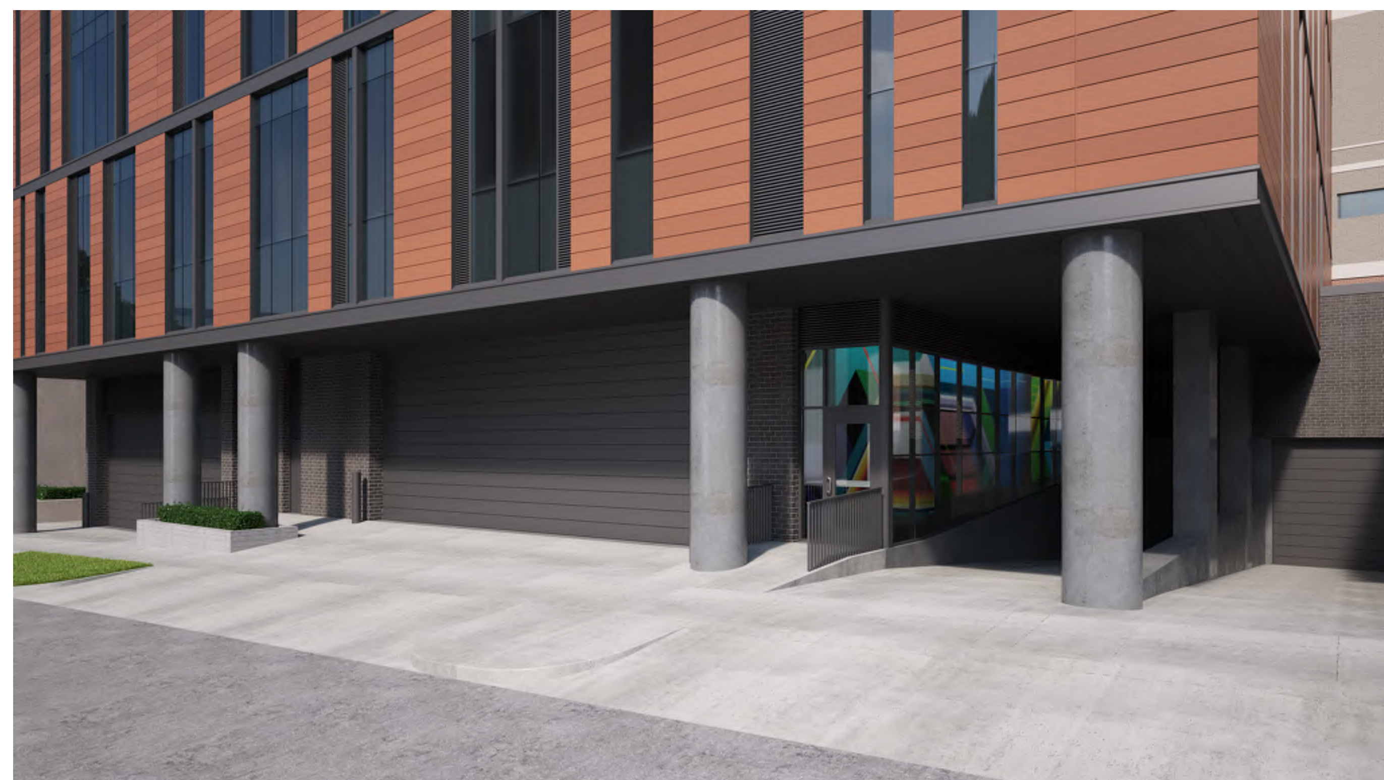
Street Level East
