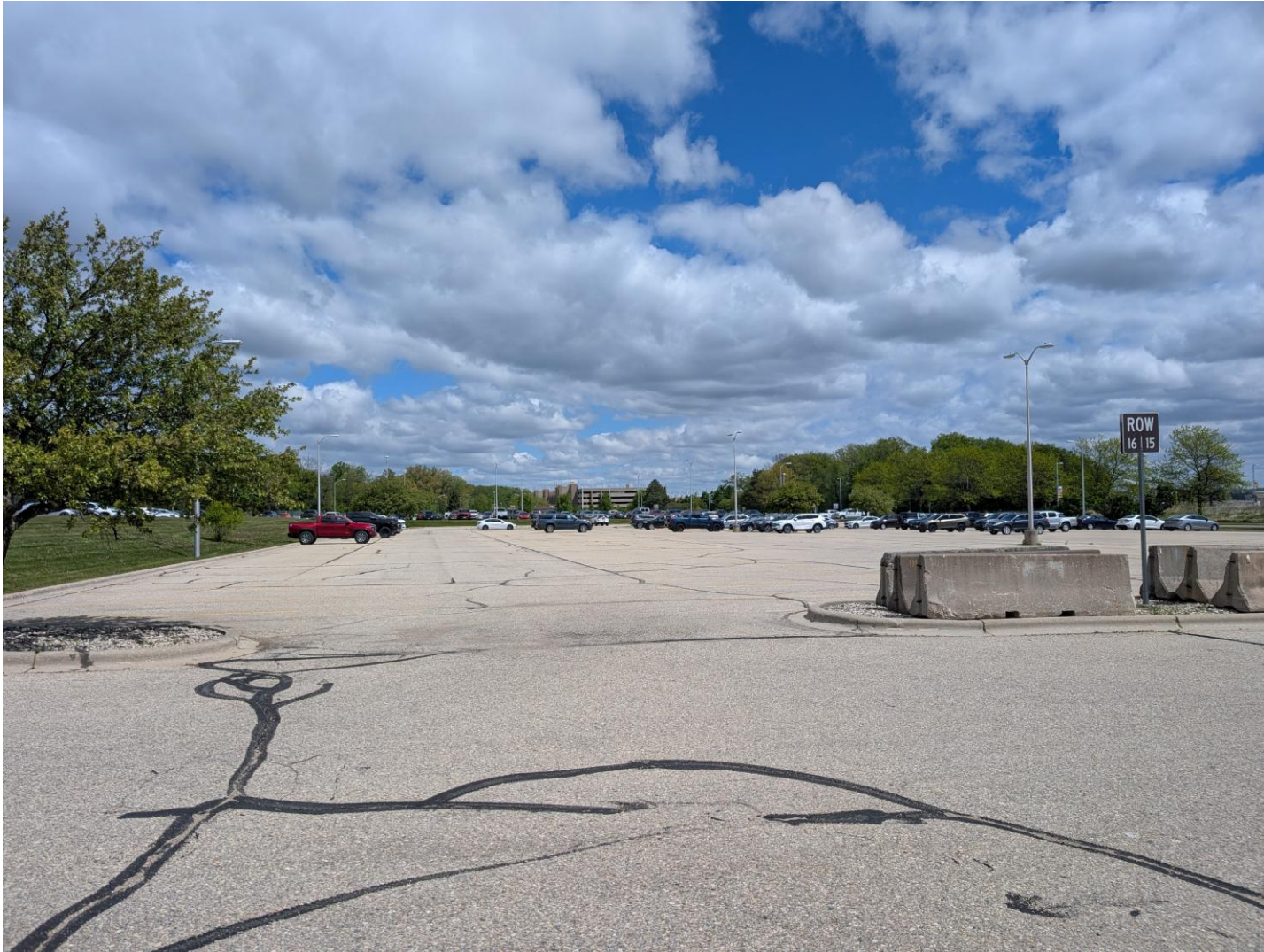
Existing Economy Parking Lot, Looking North
