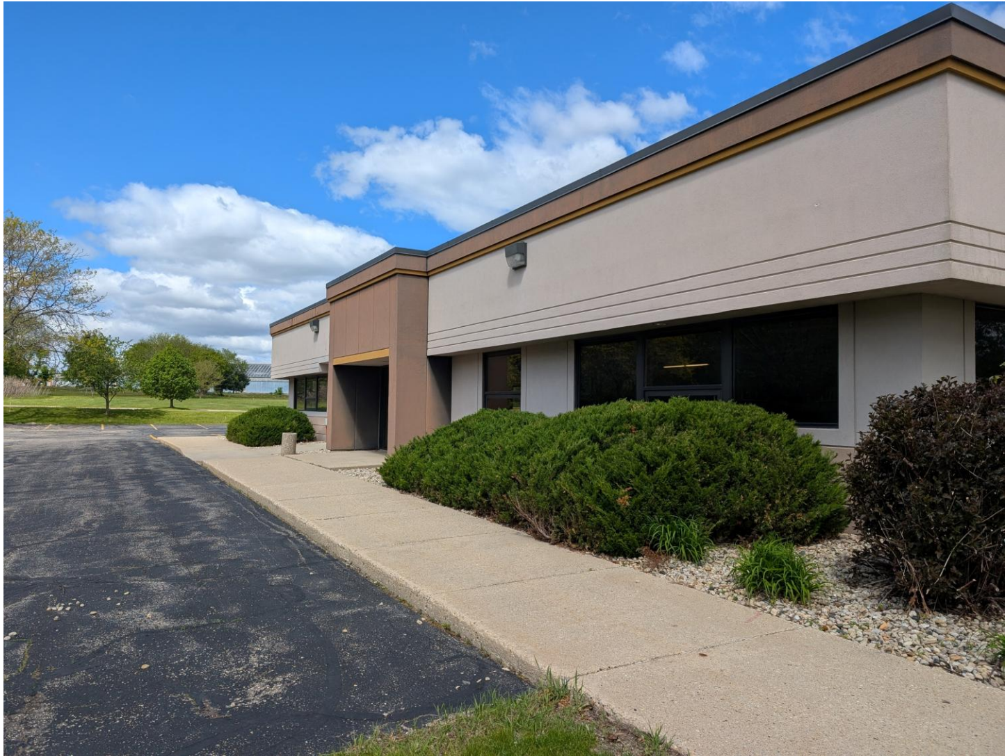
Existing Building, South Elevation
