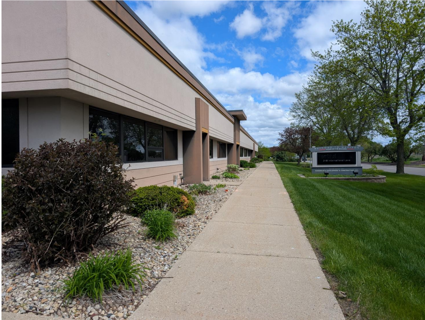
Existing Building, East Elevation
