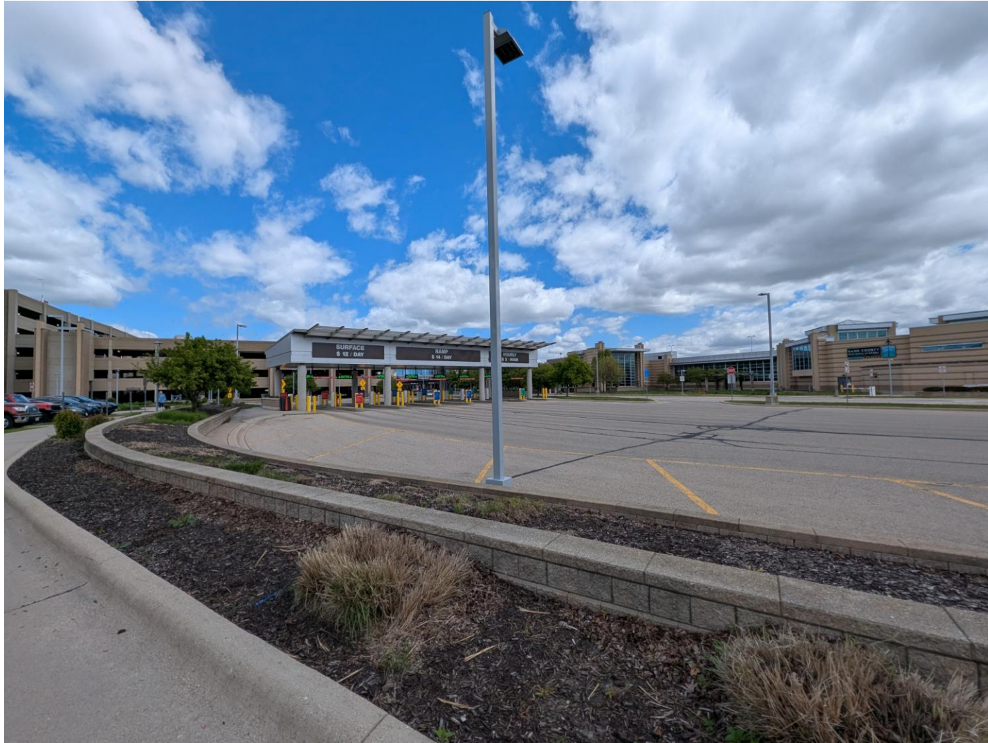
Parking Entrances, Terminal on Right
