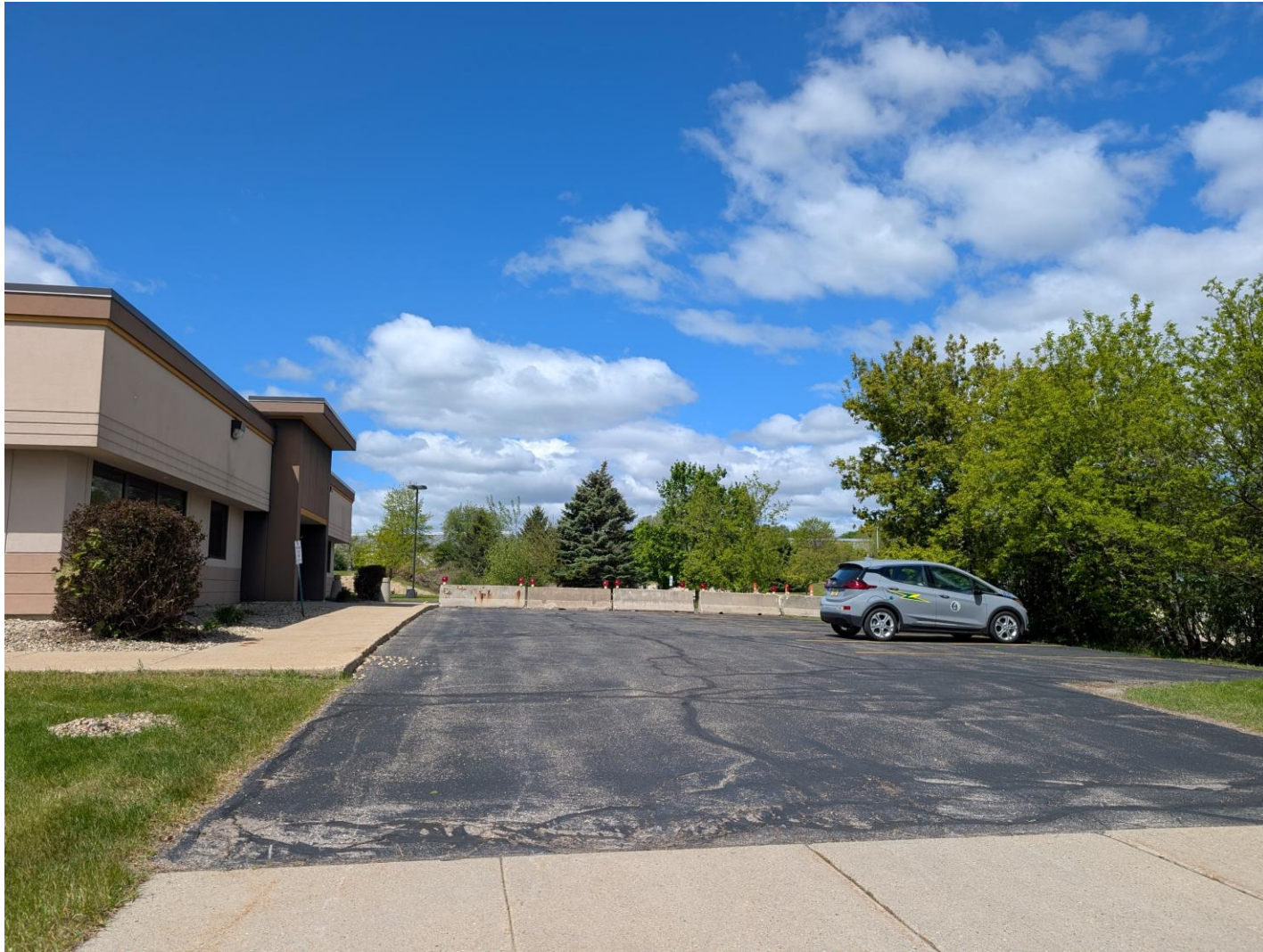
Existing Building, North Elevation, Looking West
