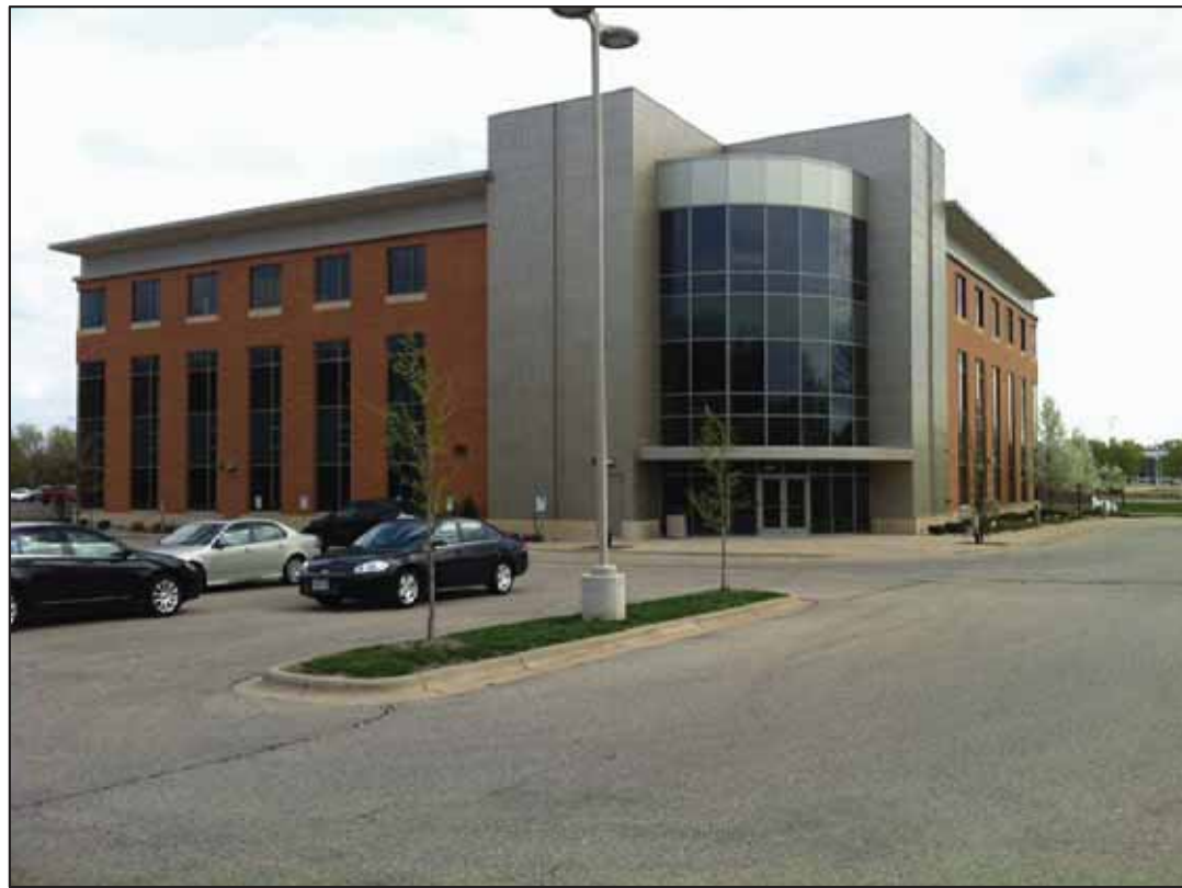
EXISTING 660 JOHN NOLEN DRIVE OFFICE BUILDING
