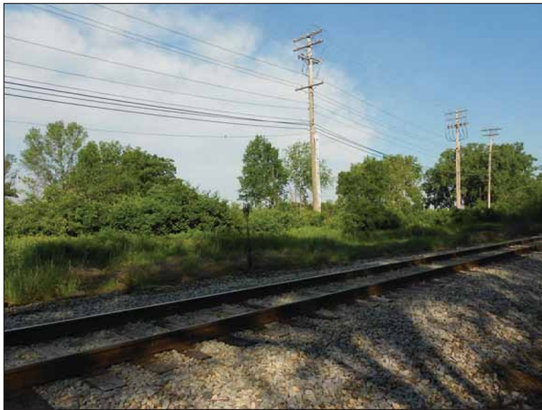
SITE LOOKING NORTH AT OVER HEAD POWER LINE
