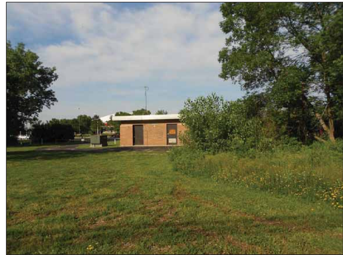
SITE LOOKING WEST AT BACK OF EXISTING PUMP HOUSE
