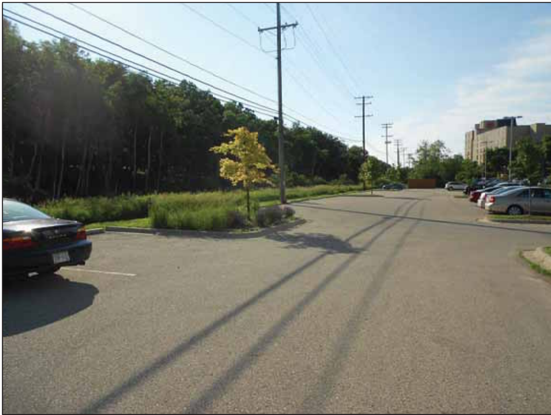
SITE LOOKING NORTH AT EXISTING PUMP HOUSE
