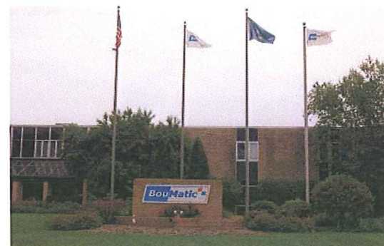
Phase 1 Opportunities: Neighbors like the facade improvements at Pelayo's (top) and the attractive landscaping at BouMatic (bottom). These examples show what can be done elsewhere in the Grid Development Area for immediate improvements.
