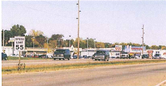
Rural Cross Section: Stoughton Road has a wide cross section typical of rural settings, with limited curb and gutter and a large central swale for drainage and lane separation.
