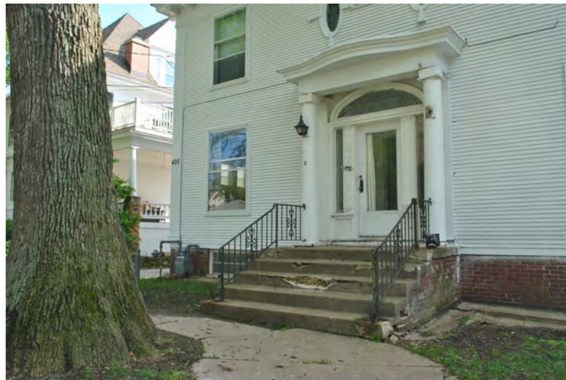
View of Front Stair
