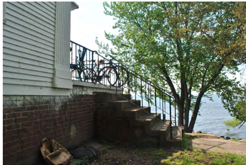
View of Porch Stair
