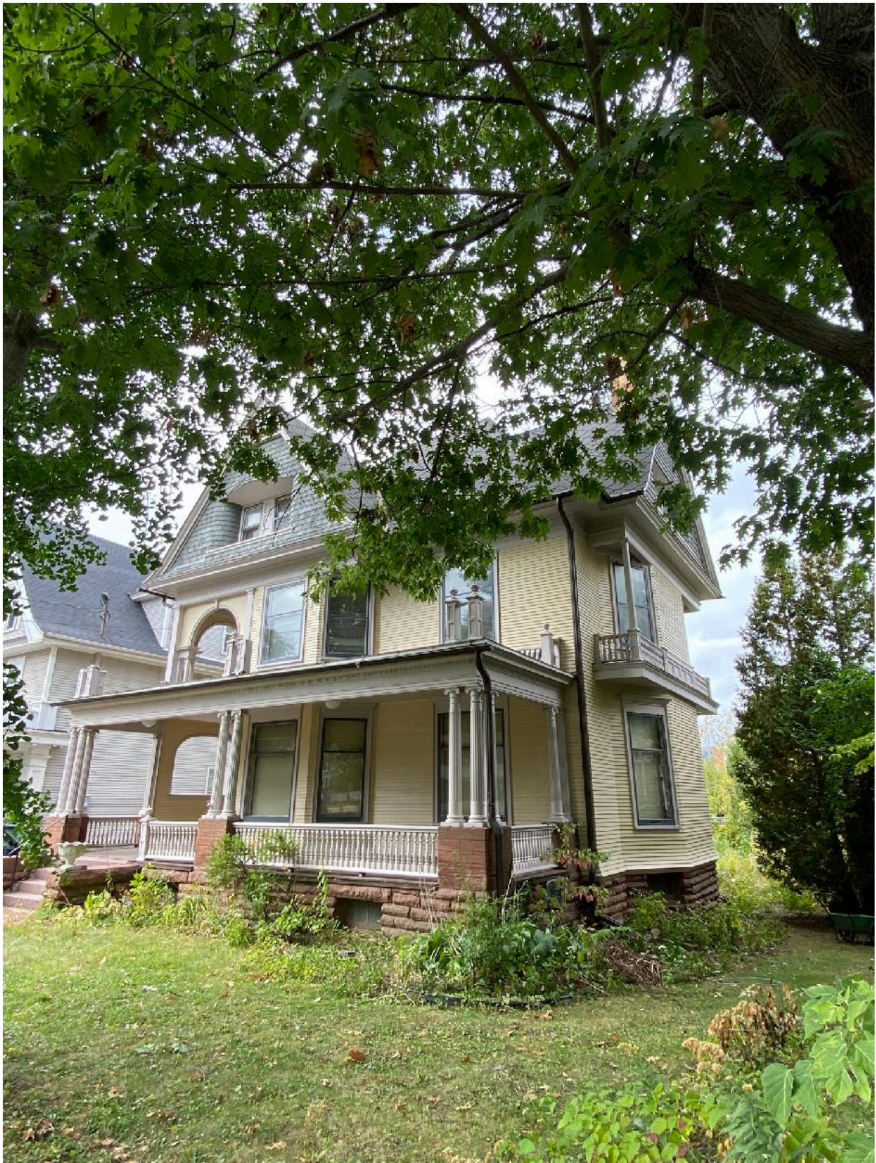
South/East Facing Elevation of 848 Jenifer Street
