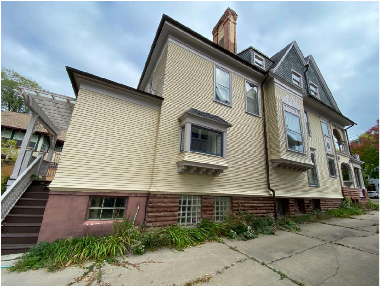
West Facing Elevation of 848 Jenifer Street
