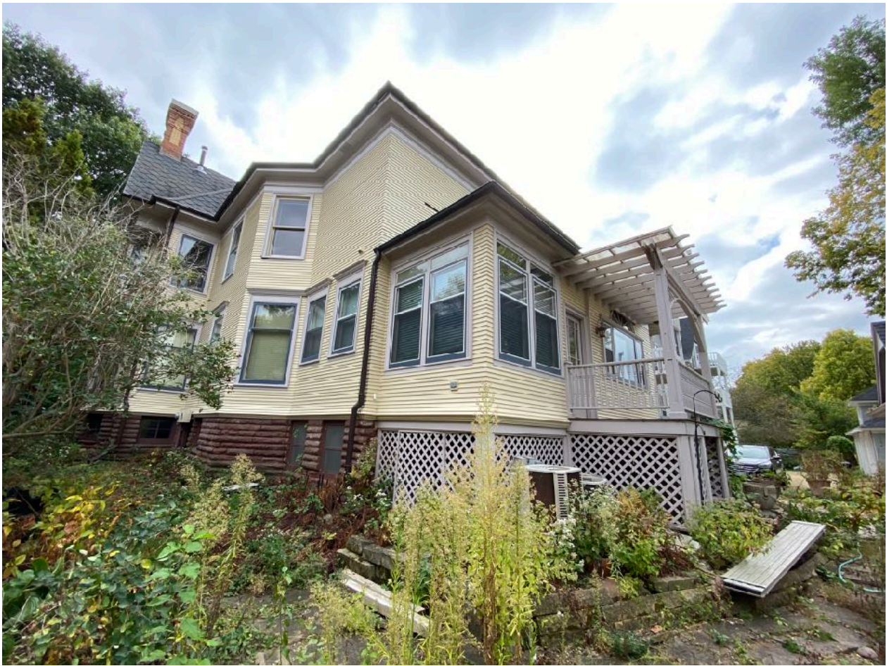
North/East Facing Elevation of 848 Jenifer Street
