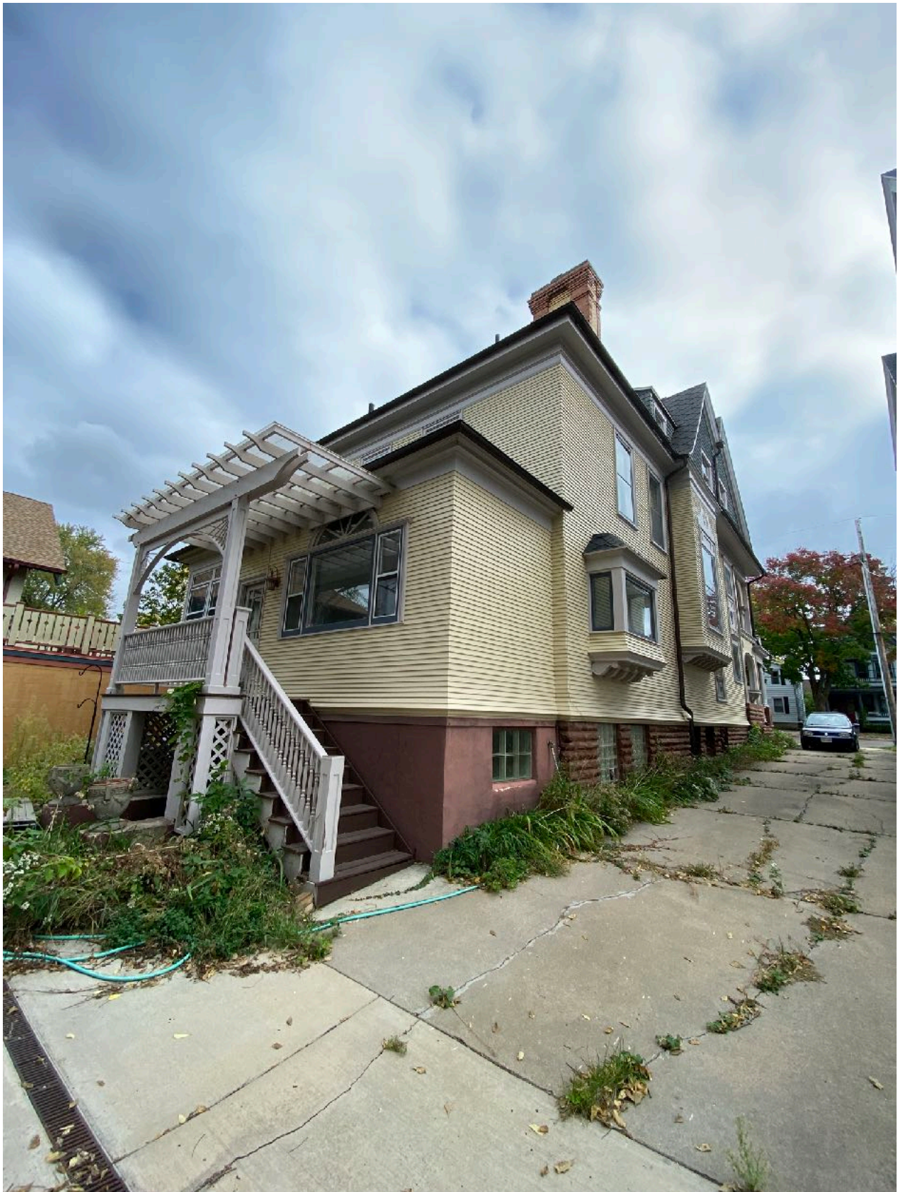
North/West Facing elevation of 848 Jenifer Street
