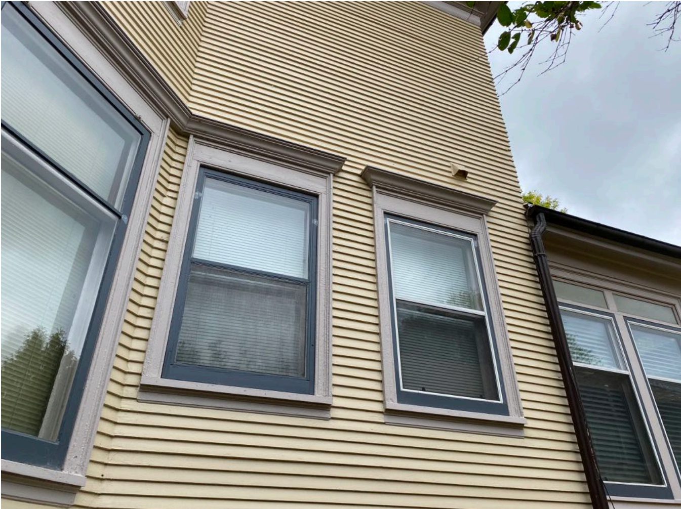
Photo of Existing Bathroom Vent on East Facade (Item 3)
