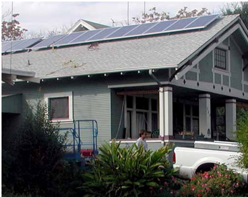
Mount collectors flush below the ridgeline on a sloping roof.
