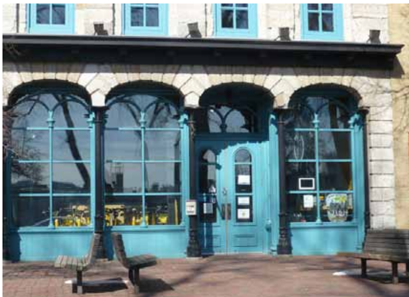
The shape of the transom is important to the proportion and character of the storefront, and it should be preserved in its historic configuration.
