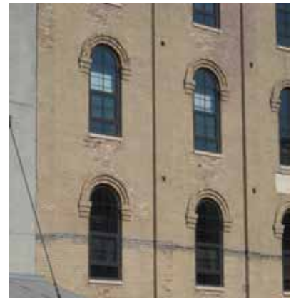
All decorative trim around a window shall be retained, including lintels, pediments, moldings or hoods.
