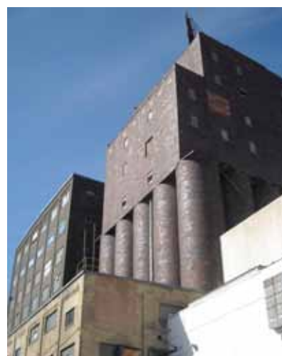
The Water Power Area contains a diversity of building heights that reflect the functional needs of the buildings. The grain elevators extended upward out of the mid-level height of the milling, warehousing, and industrial buildings.
