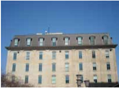
The character of a historic roof should be preserved, including its form, roof pitch, orientation, overhang and materials.
