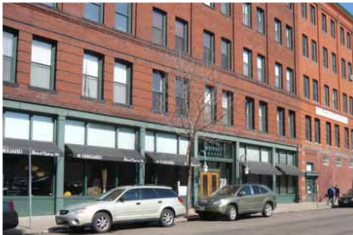
Warehouses were typically oriented to the street and rail yards resulting in a double-fronted building. Preserve platforms and entrances that occur on both sides of these building types.
