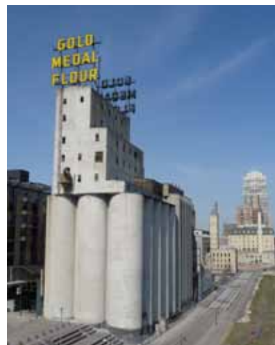
The massing of buildings within the Water Power Area reflects the needs for which the buildings were designed.
