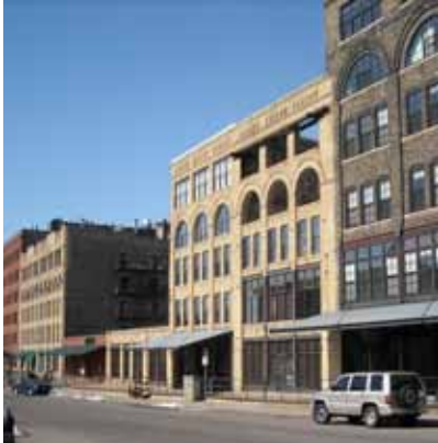
The design effect of recessed openings, projecting moldings and material change promotes a composition of light and shadow along the historic building facade that can be recognized along the street.
