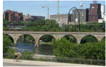
The Stone Arch Bridge is a key feature in the district. It is also a great example of a successful adaptation of a RR bridge to a multimodal path.
