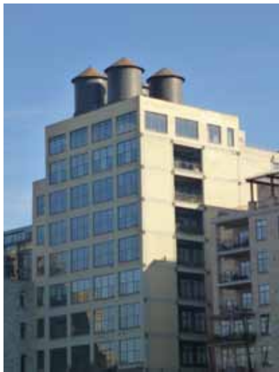
Preserve significant stylistic and architectural features, including roof-top elements.
