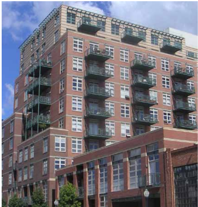
Arrange windows to reflect the traditional rhythm and general alignment of windows in the area.
