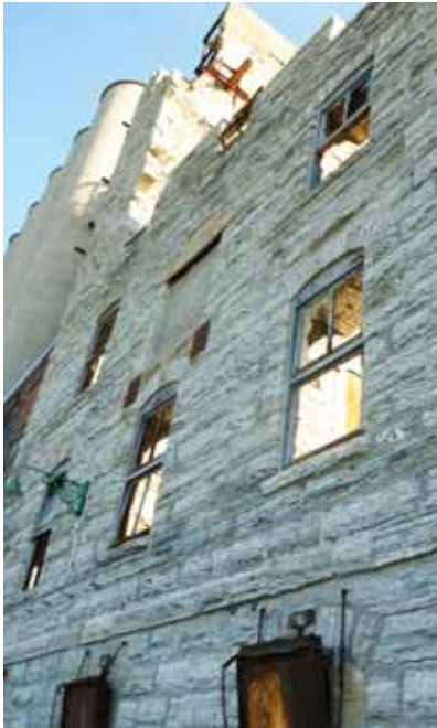
Preserve original building materials.
