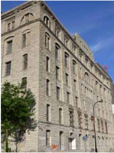
Preserve significant masonry features.
