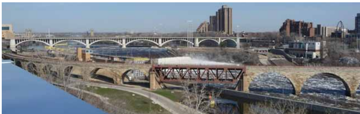
View of the Water Power Character Area from the Guthrie Theater
