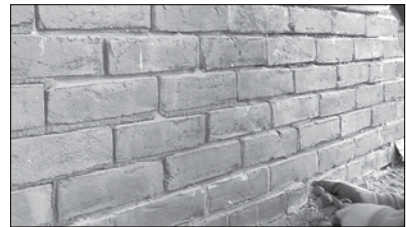
Tool and repoint mortar joints where there is evidence of deterioration.
