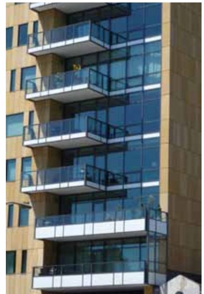
The balcony should appear mostly transparent. Simple metal work is most appropriate on mixed-use and residential mid- and high-rise buildings.
