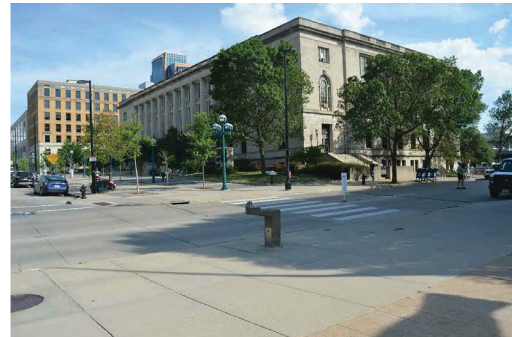
V1 - Madison Municipal Building from the Southwest
