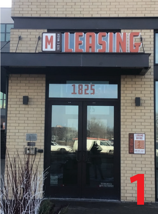
The Marling Leasing Office
