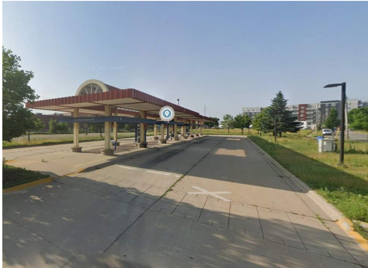
VIEW FROM NORTH TO SOUTH
