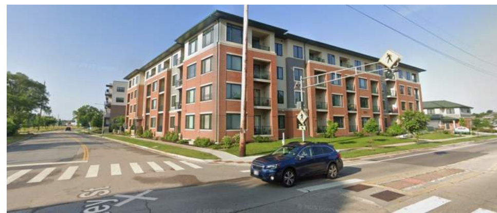
North West of Site Huxley and Aberg Ave Intersection
