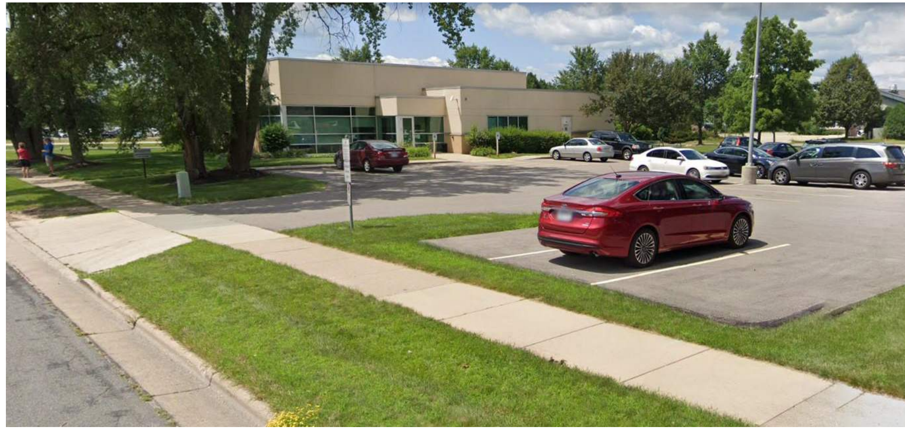
NORTH STOUGHTON HEALTH CENTER
