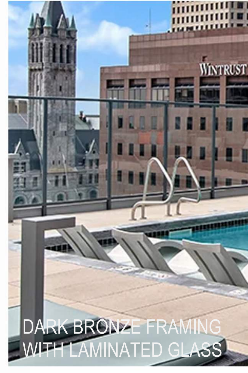
GLASS GUARDRAIL ASSEMBLY
