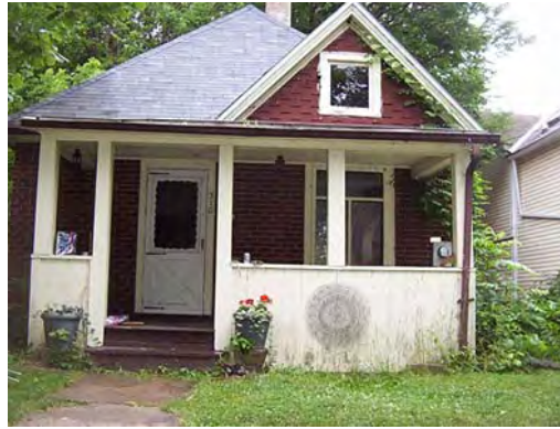
310 S. Baldwin St.(removed & recycled)
