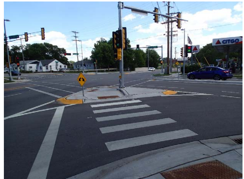
Continental crosswalk at Fair Oaks/Milwaukee Street intersection
