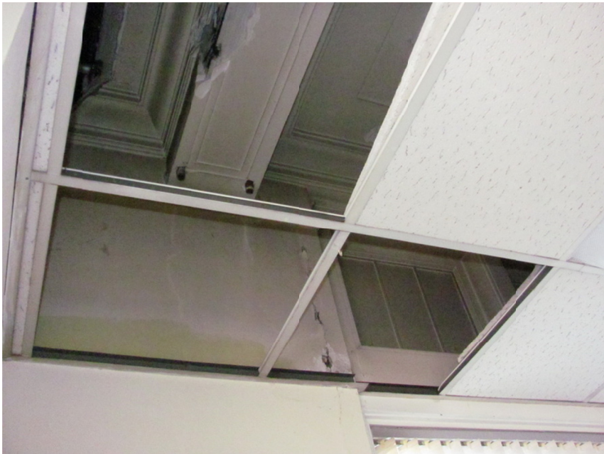
Figure 9. The original plaster ceiling and cornice are present above the suspended acoustical ceiling system. Also note the original transoms at the first floor storefront.
