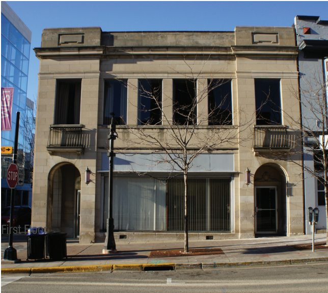
View of Front Facade
