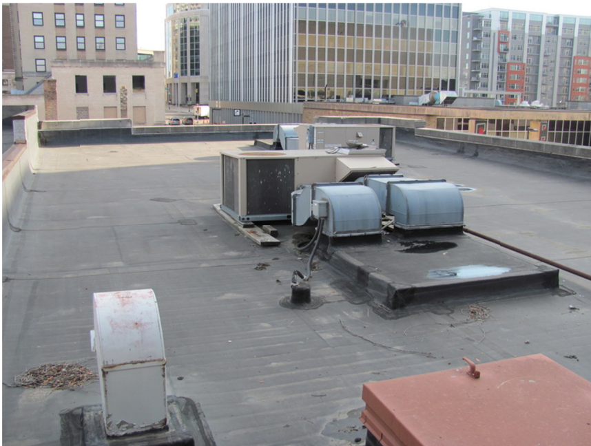
Figure 7. Overview of the roof.
