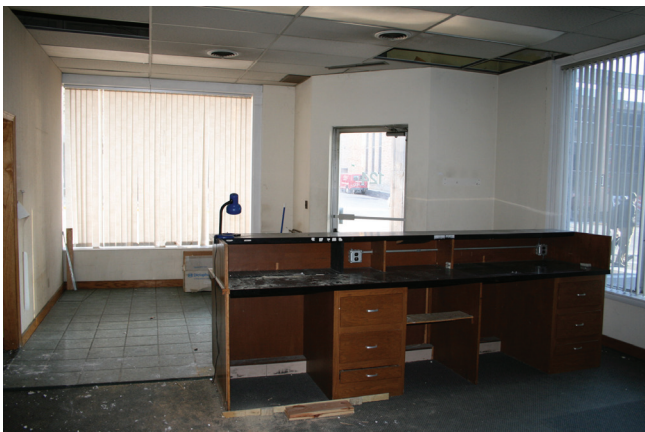
First Floor: View toward entry at corner of West Mifflin Street and North Fairchild Street
