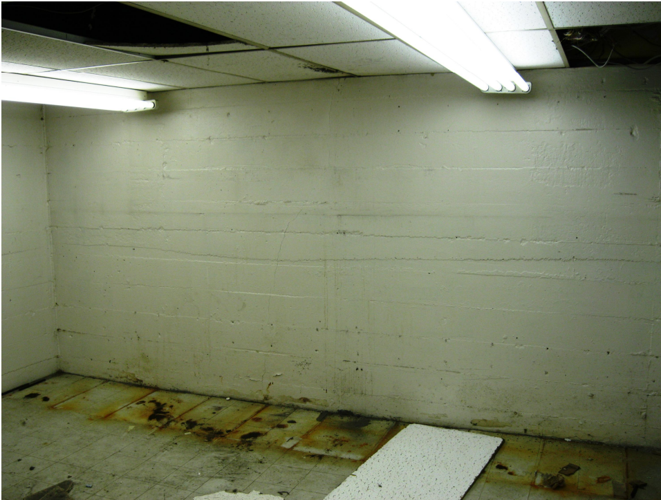
Photo 1 – Concrete basement wall at Mifflin / Fairchild corner
