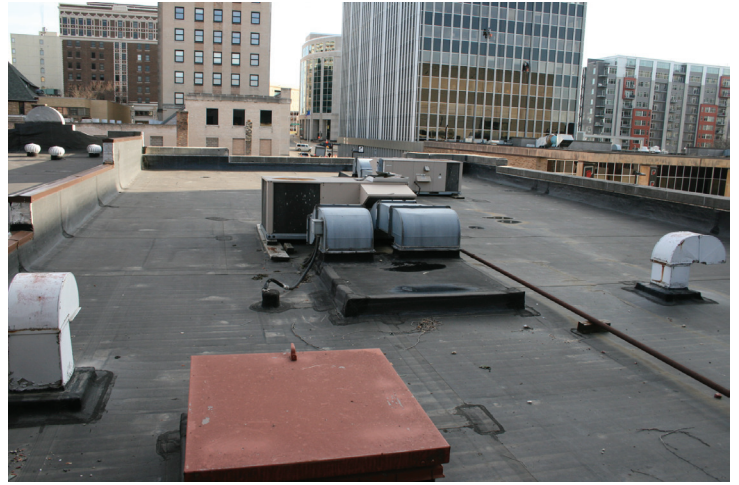
View of Roof
