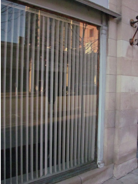
Figure 6. The storefront facing Mifflin Street has a bronze frame and fluted bronze pilasters as window jambs.
