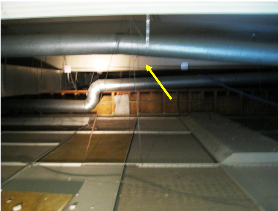
Photo 2 – Typical steel girder (encased) supporting 2 nd floor wood joists
