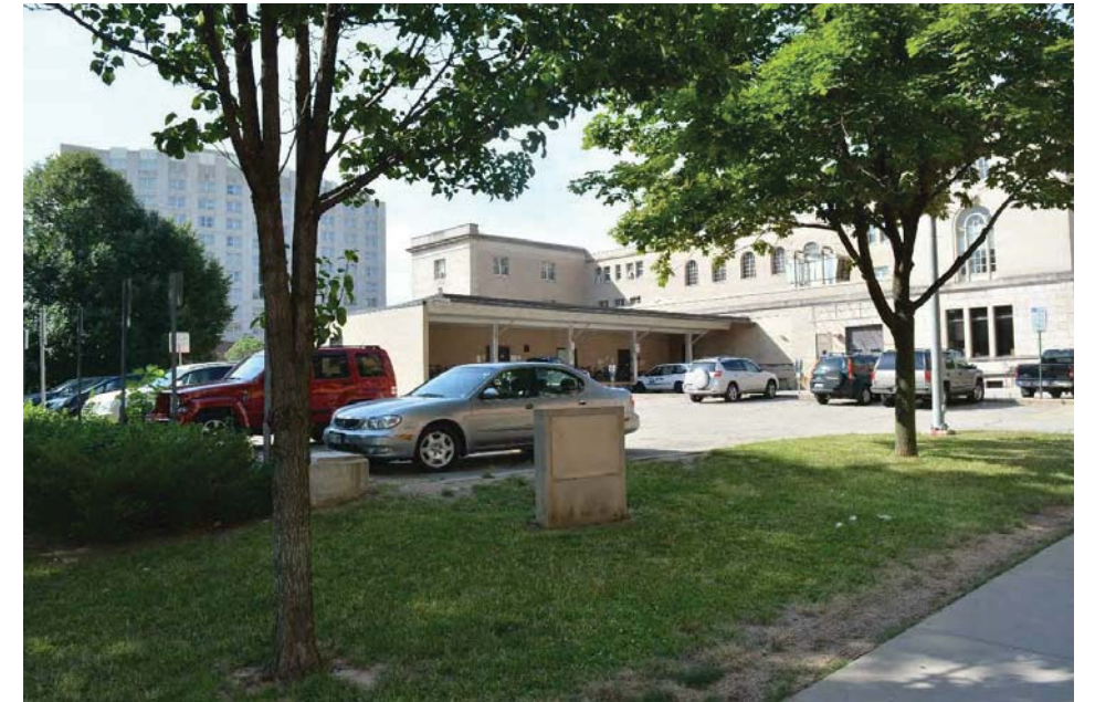
V11 - Existing site & MMB from the Pinckney & Doty intersection
