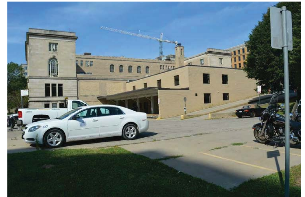
V6 - Existing site & MMB from Pinckney Street
