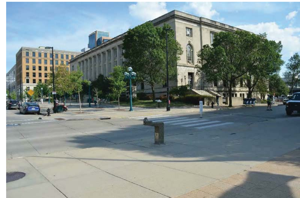
V1 - Madison Municipal Building from the Southwest
