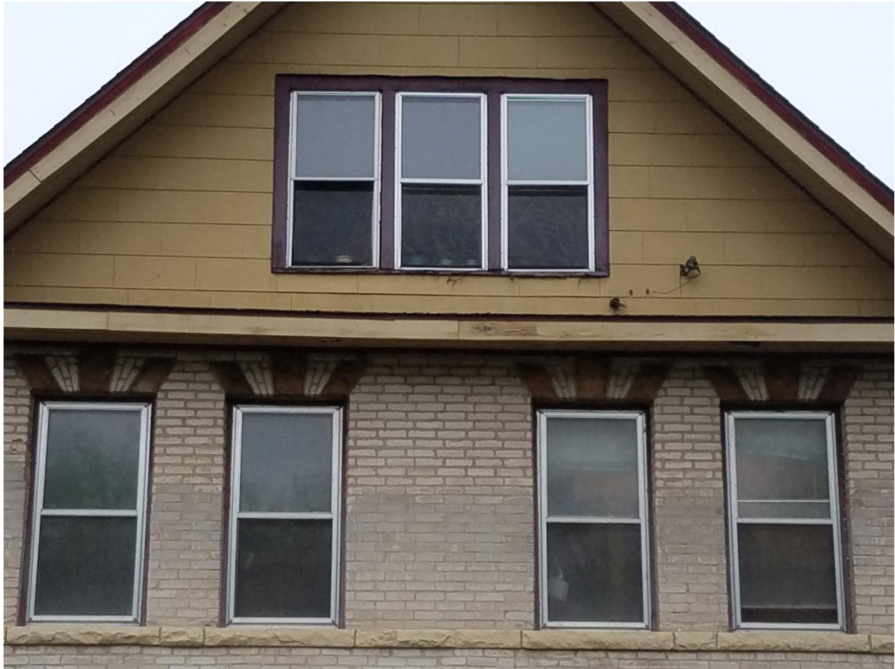
This is the front facing windows at 1014 Williamson Street.
