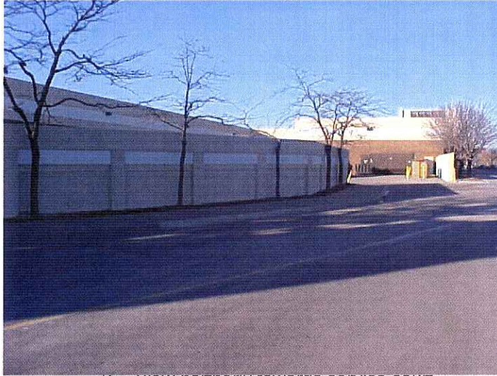
2. view northerly towards service court.
