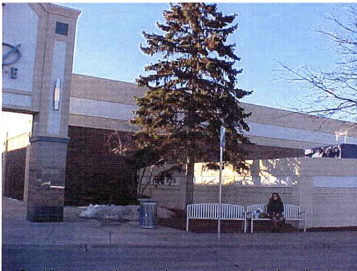
3. View westerly towards service court and mall entrance.
