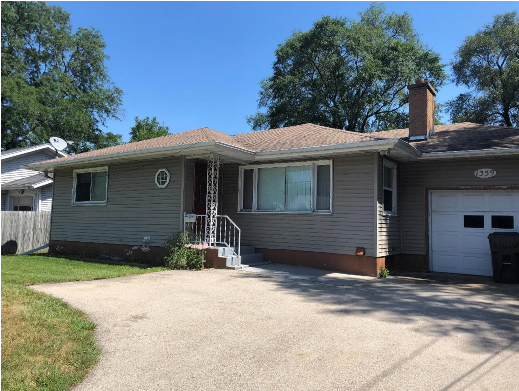
Exterior (West Side)
