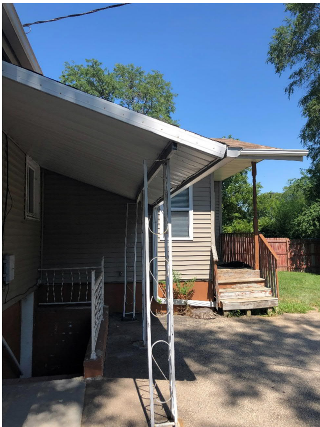
Basement stairs and canopy
