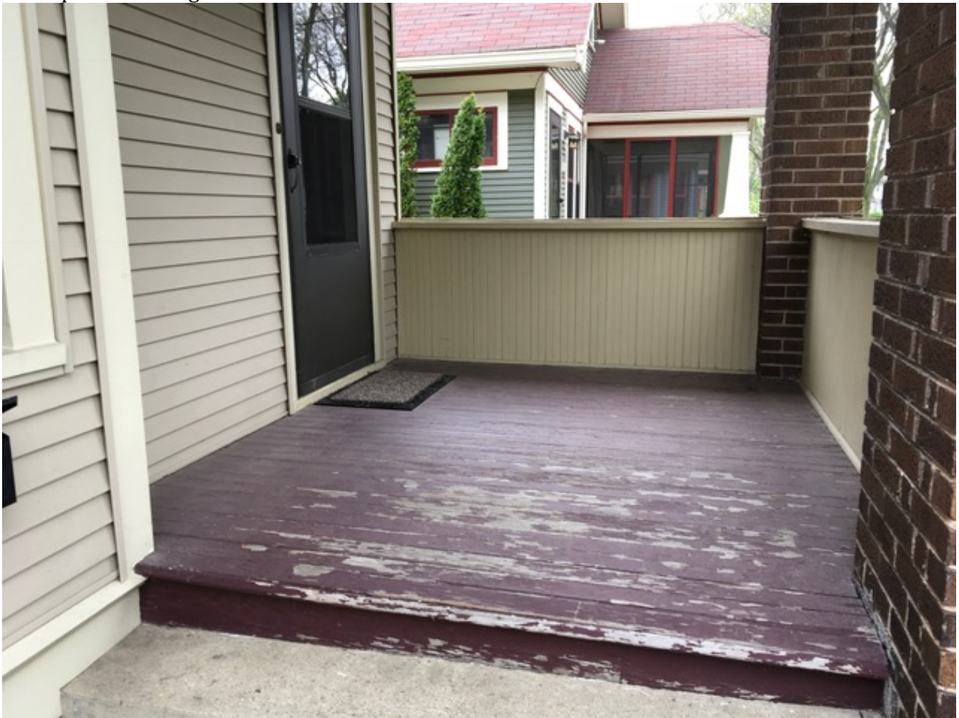
Knee wall board to be replaced
