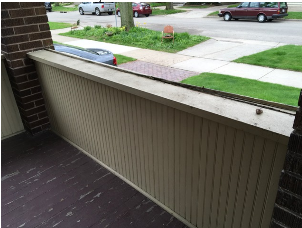
Knee wall board to be replaced
