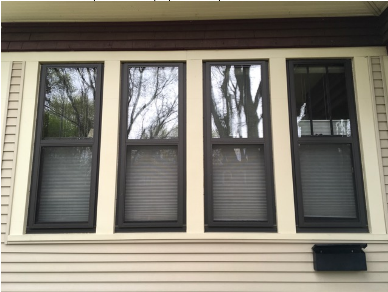
Closer view of front façade windows proposed for replacement
