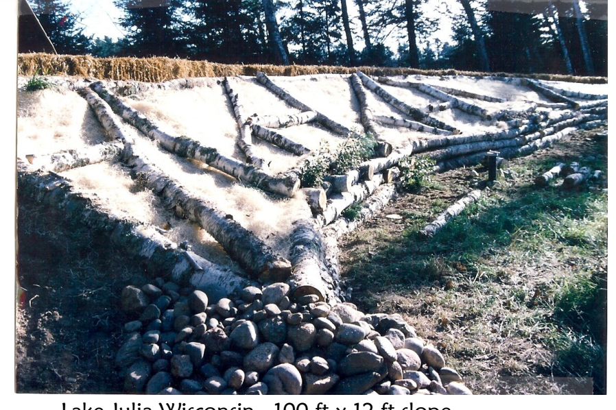
Lake Julia Wisconsin 100 ft x 12 ft slope Stabilized and restored with Birch logs & limbs
