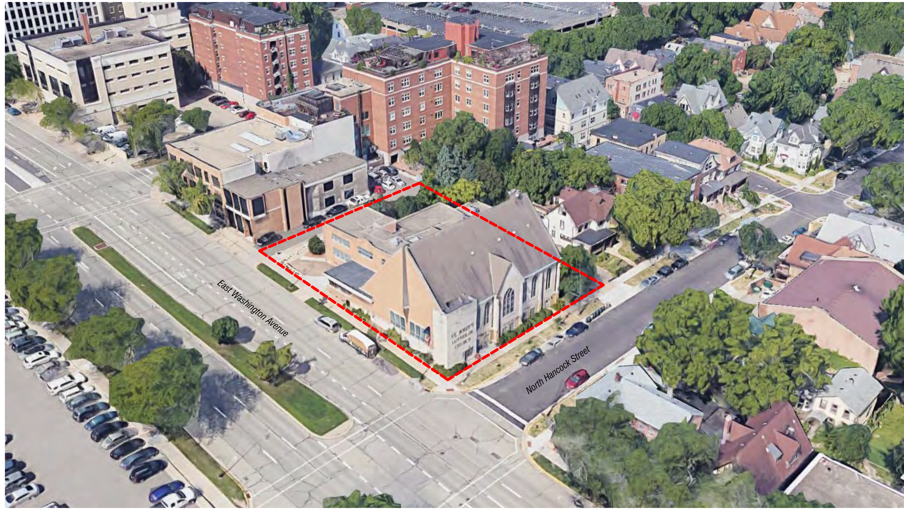
332 East Washington Avenue - Existing Site
