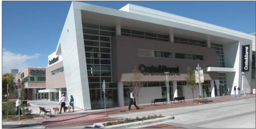
Cherry Creek North Redevelopment | Denver, CO
