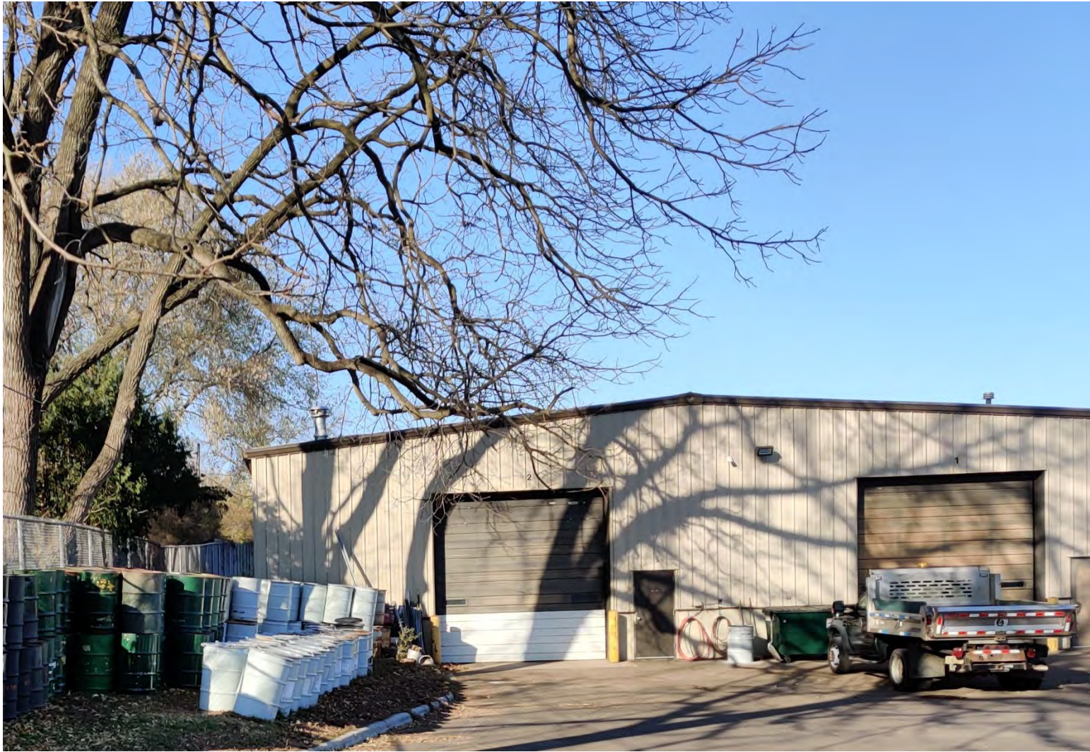
M-5 Outside Vehicle Wash Area
