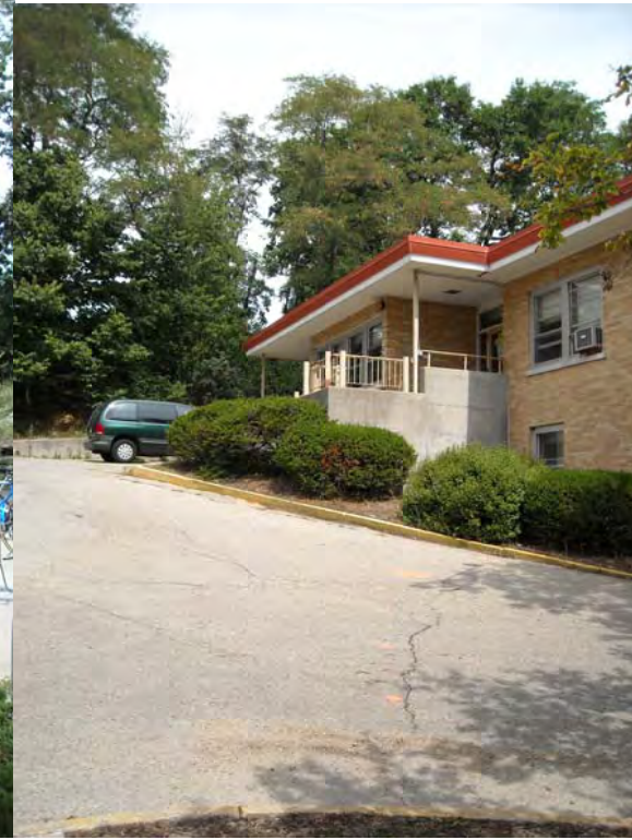
Fire lane will extend from here to rear of addition.
