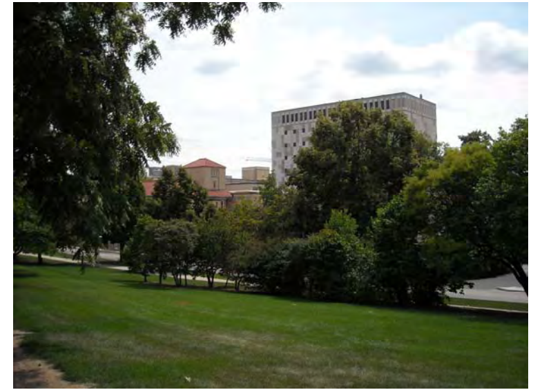
Vegetation to be removed by garage entrance.
