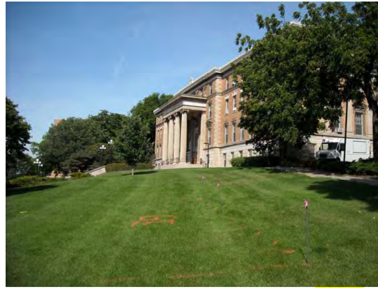
Upper extent of garage entrance in orange. Garage entrance will extend 8' above land surface at this point.
