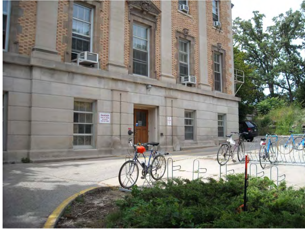
Post showing southwestern corner of addition. Fire lane to extend between addition and Ag Hall.
