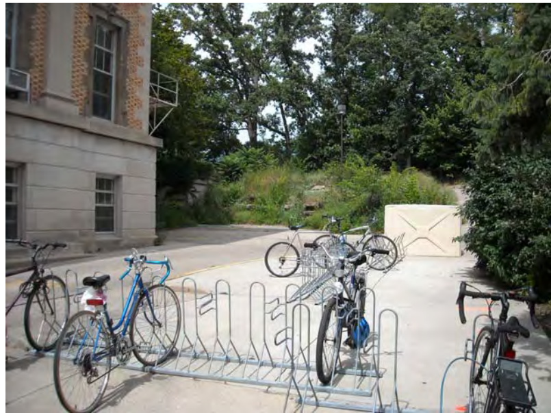
Western extent of addition, in orange, looking north.
