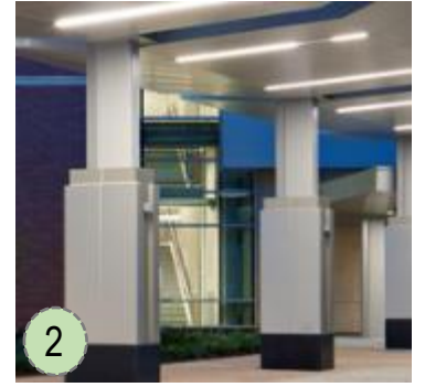
2 Painted Structural Columns with Metal Panel Base Wraps
