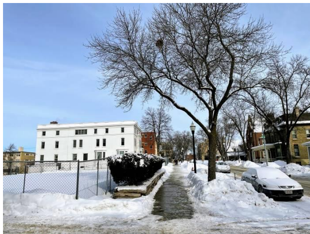
126-140 Langdon St. Facing Southeast from the northwest corner of the site.
