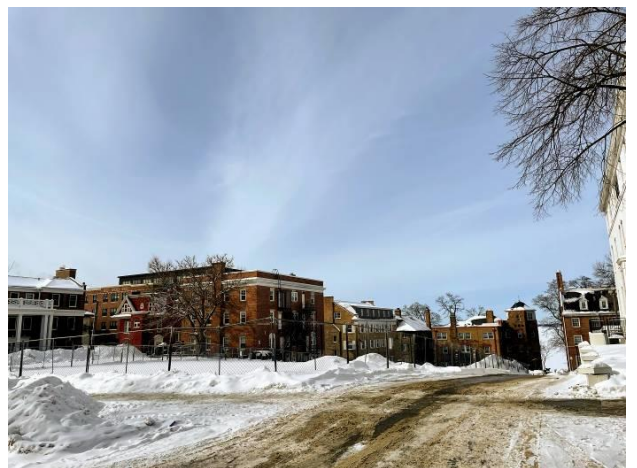
126-140 Langdon St. Facing Northwest from the Langdon St. across the site.
