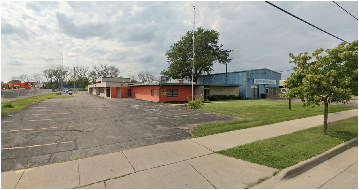
Adjacent site to North
