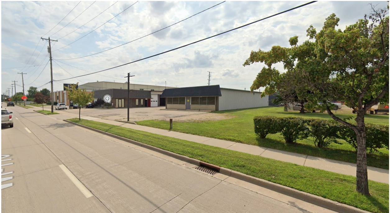
Adjacent Site to South
