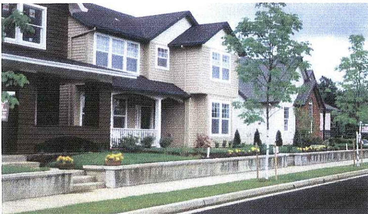
Single family homes, Fairview Village, Fairview
