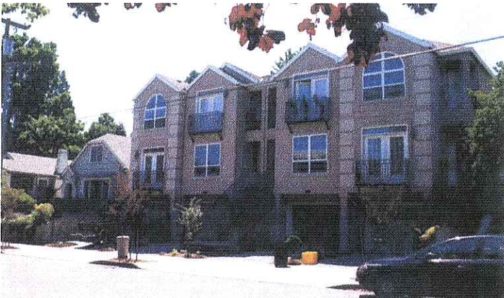
Townhomes, Northwest Portland
