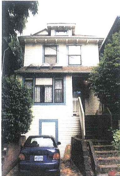
Duplex, Southeast Portland
