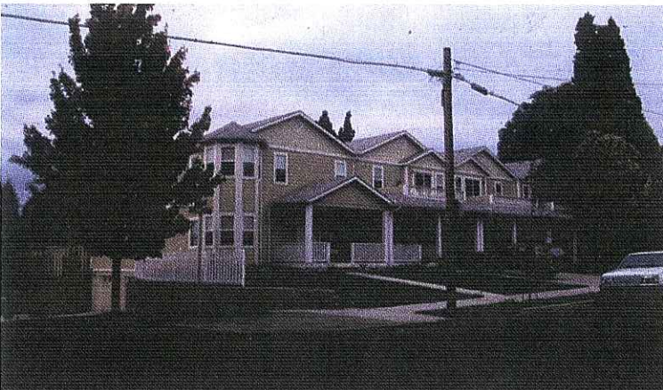
Infill rowhomes Southeast Portland
